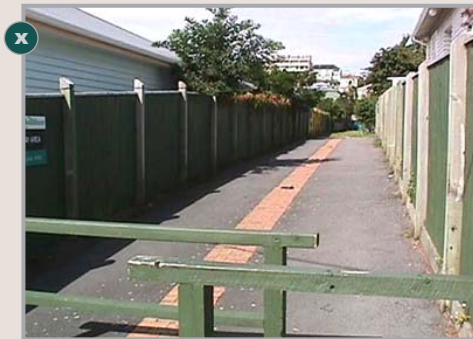
Narrow access to back-section park - security risk.
