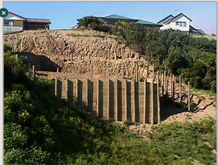
Difficult site access and costly building platform construction.
